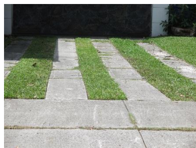
4.2 Concrete Wheel Strips
