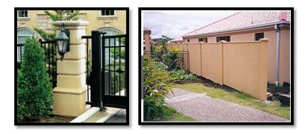
**Pilaster.** An engaged pier or pillar, often with capital and base; decorative features that imitate engaged piers but are not supporting structures, such as a rectangular or semicircular member used as a simulated pillar in entrances and other door openings and fireplace mantels. A pilaster often contains a base, shaft, and capital and may be constructed as a projection of the wall itself.
