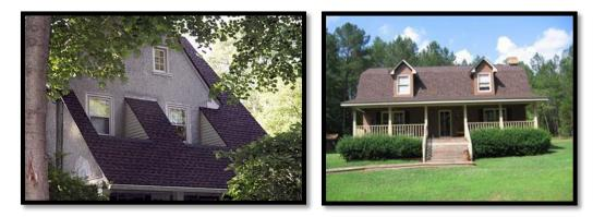
*Side-Gabled Roof.* A gable whose face is on one side (or part of one side) of a house, perpendicular to the façade. (See Section 3.2: Roofs)
