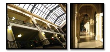
**Arch.** A curved construction which spans an opening; usually consists of wedge-shaped blocks called voussoirs, or a curved or pointed structural member which is supported at the sides or ends. Arches vary in shape from the horizontal flat arch through semicircular and semielliptical arches to bluntly or acutely pointed arches.
