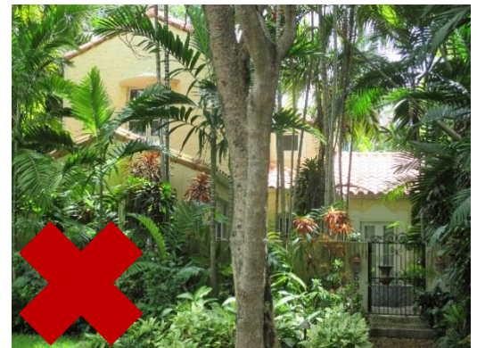
4.12 Overgrown plants obscuring the front facade
