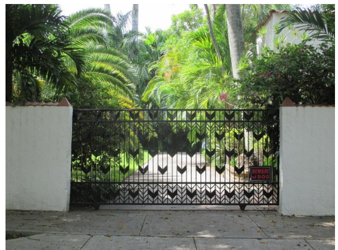
FIGURE 4.5 Gate with at least 60% visibility with design and color complementary to historic home
