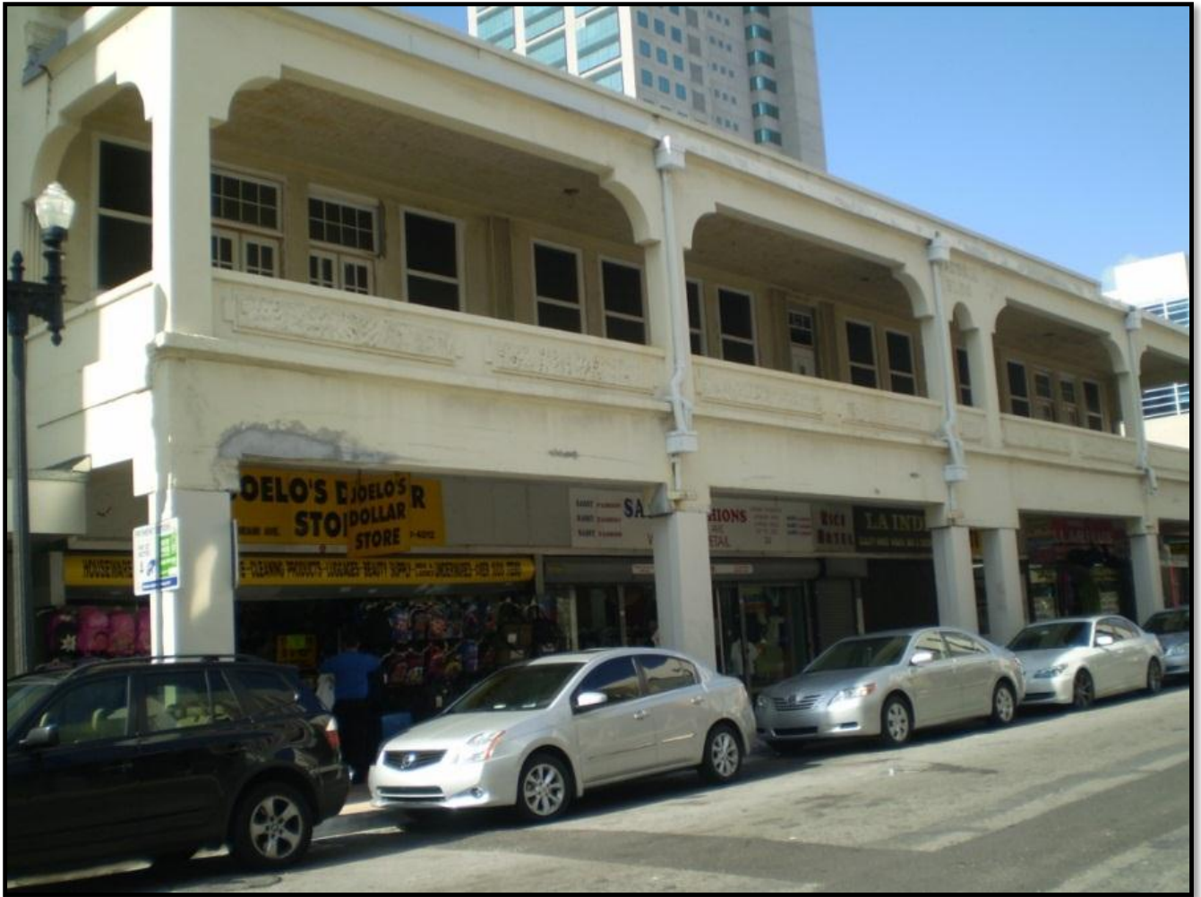
2.3 Waddell Building, 24 N Miami Avenue, Built 1916
