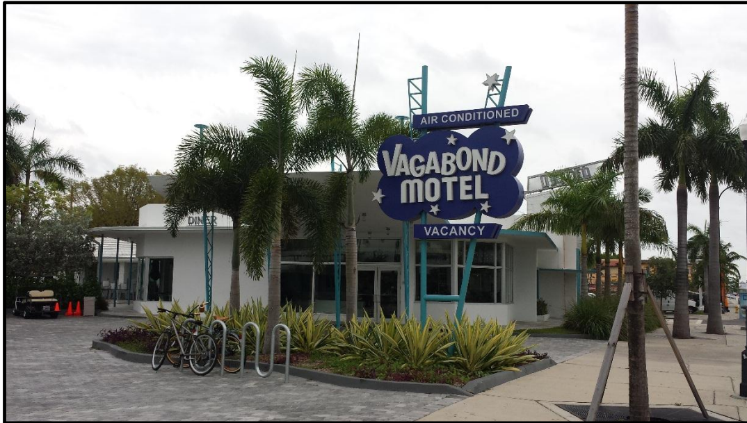
2.14 The Vagabond Motel, 7301 Biscayne Boulevard, Built 1953
